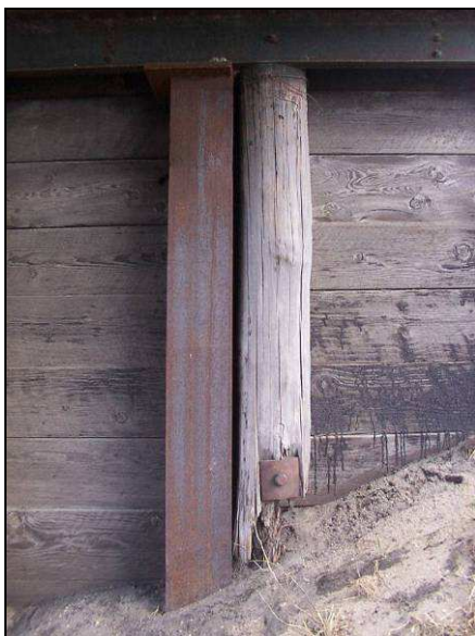
FIG. 4.3 — New steel pile driven adjacent to a defective timber pile
