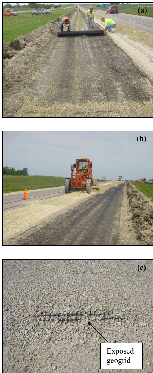
FIG. 2.15 — Geogrid stabilization (a) rolling the BX1200 geogrid over the soft subgrade layer (b) spreading crushed limestone over the geogrid (c) exposed BX1200 geogrid at about 2.4 from the pavement edge after 10 months
