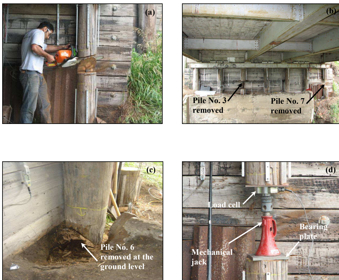
FIG. 5.7 — Destructive static load tests (a) removing pile No. 7 (b) a section from pile Nos. 3 and 7 removed (c) a section near the ground level is removed from pile No. 6 (d) mechanical jack and load cell used to restore the dead load carried by pile No. 7
