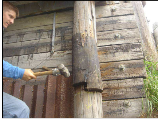
FIG. 5.10 — Repairing pile No. 7 using the splicing technique
